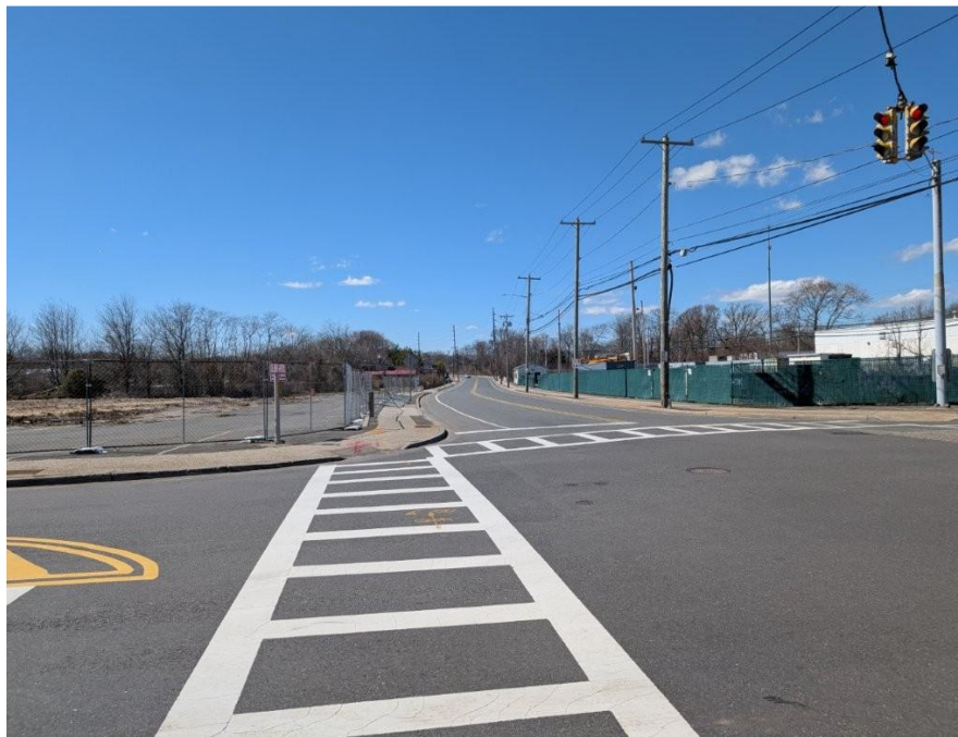
View West along Division Street, Frontage
